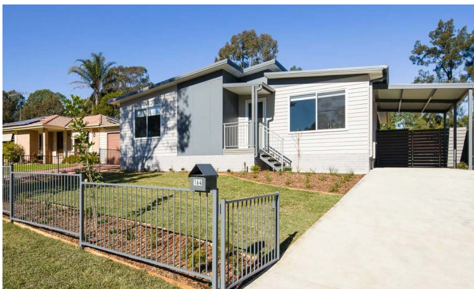
AHO property with cement clad and brick dwarf wall around footings.
