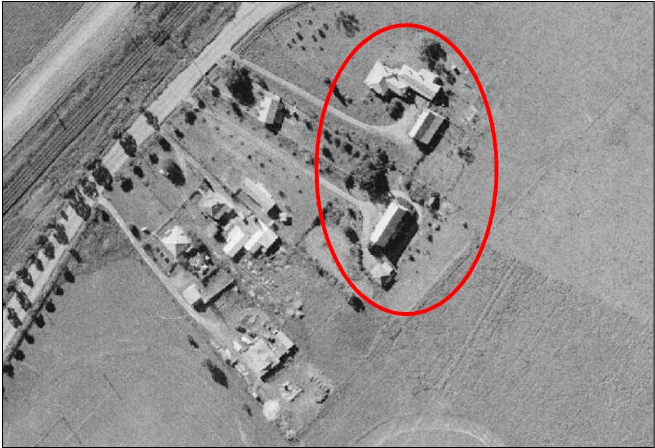
Figure 11: 1961 aerial view of the Warby homestead, Stables and Barn (source: GBA Heritage Peer Review)
