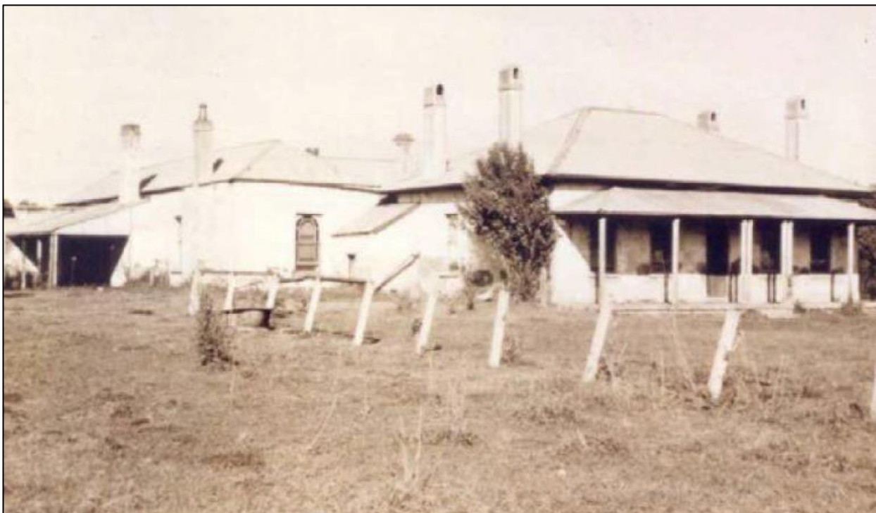
Photo 4 - Former Warby homestead (Leumeah House) (source: GBA Heritage Peer Review)
