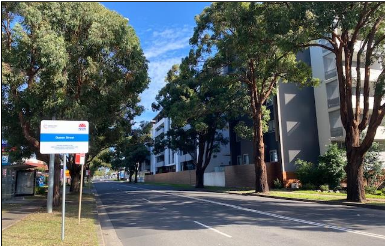
Photo 2: View looking south along Queen Street from the front of the site.
