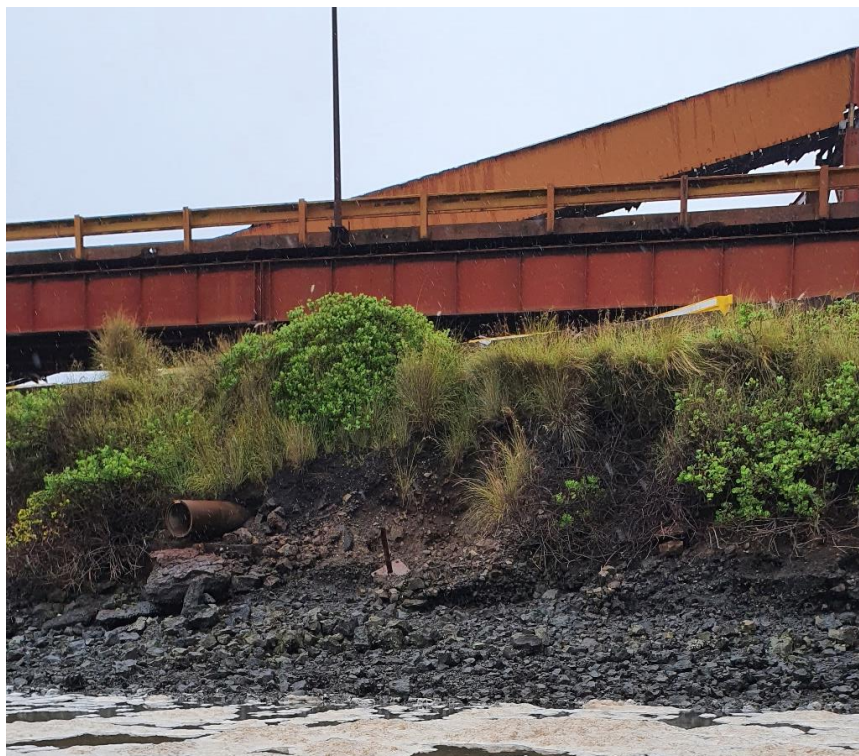
Figure 6: General Condition of Embankment – Starting to Undermine Road
