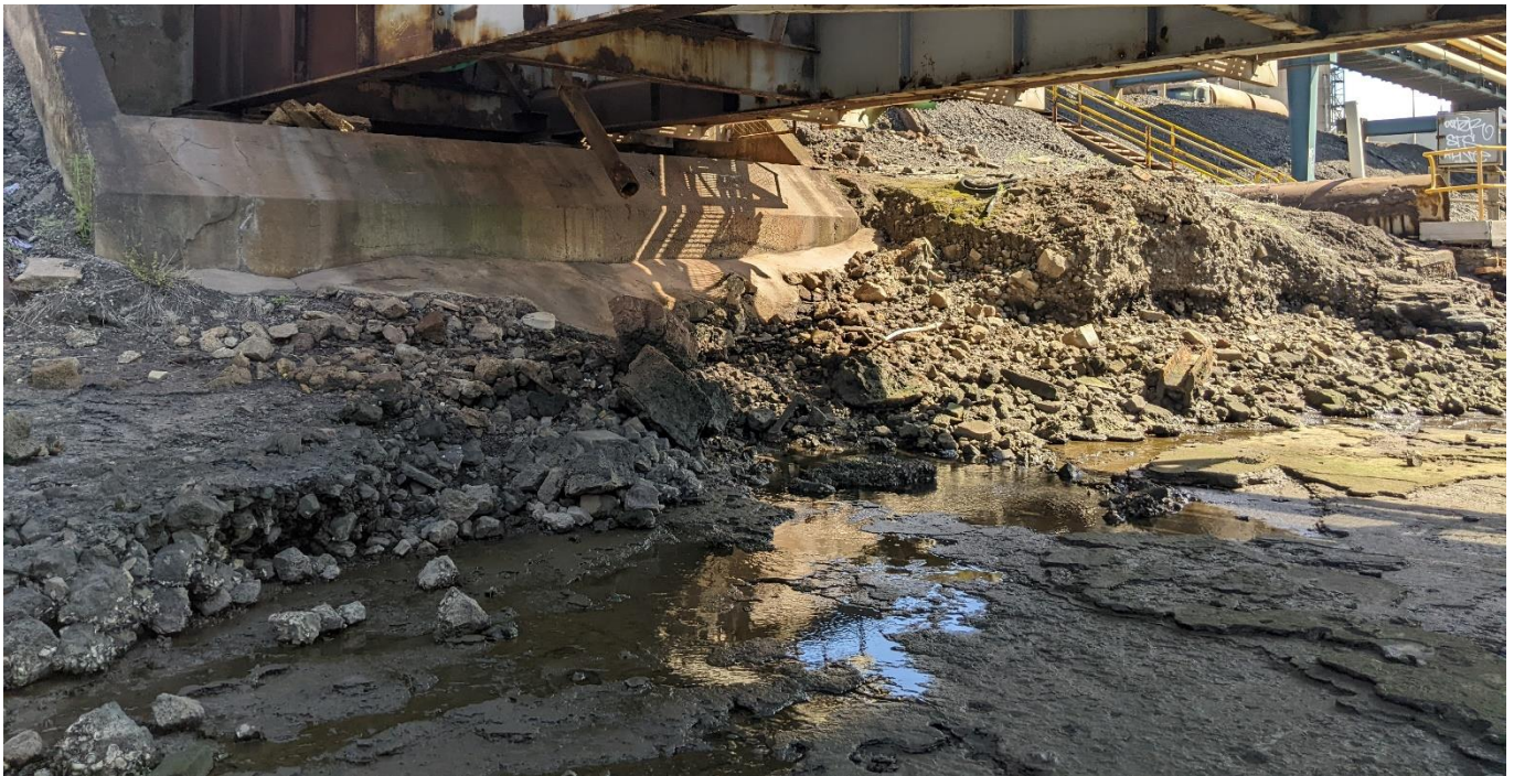
Figure 5: Erosion of Bank under Bridges (Low Tide)
