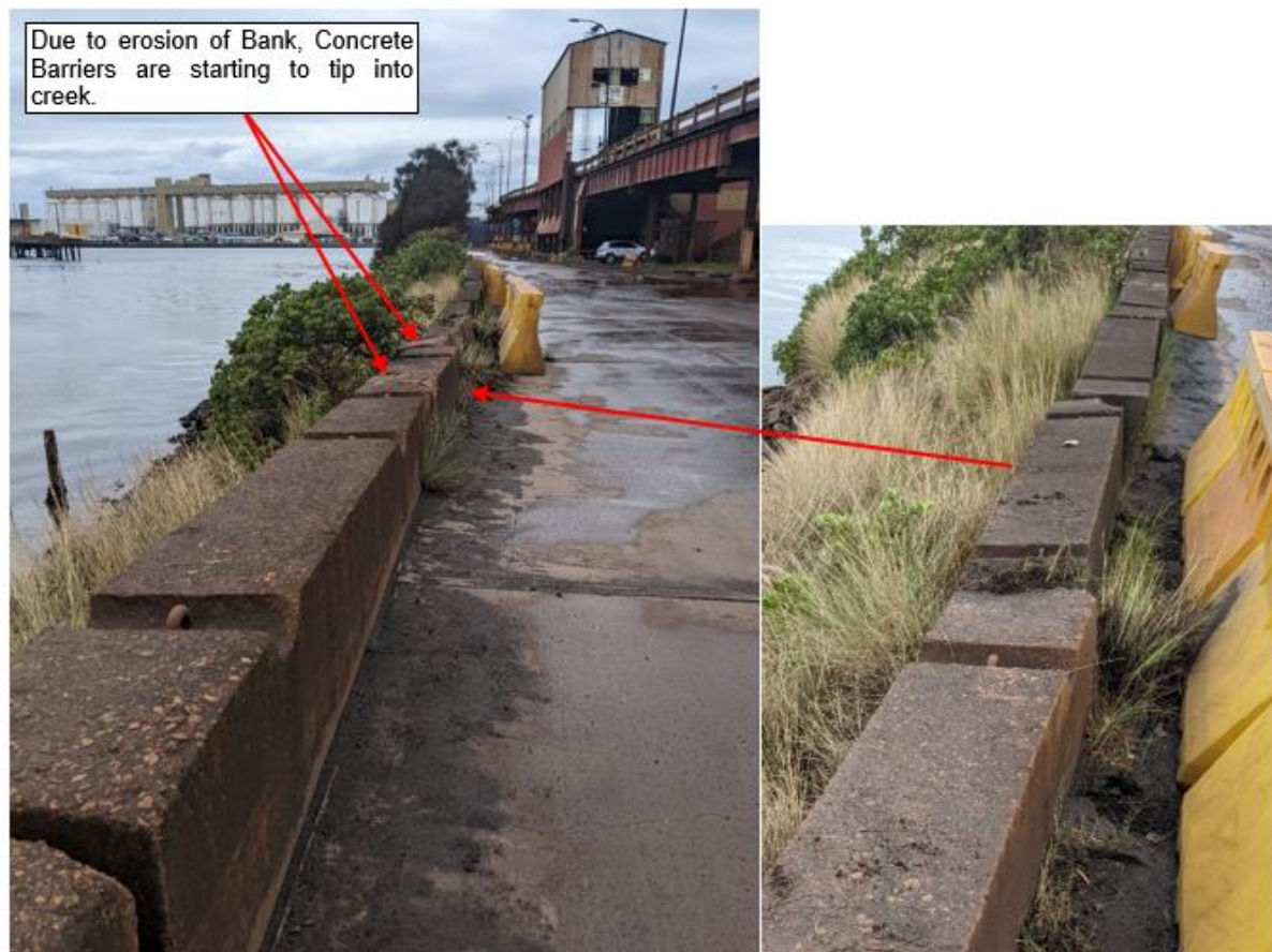
Figure 7: General Gradient of Embankment - Starting to Undermine Road
