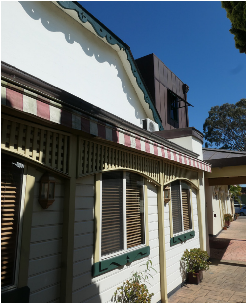
Figure 3.9 Undated addition to the east side of Collaroy House, probably replacing an original verandah
