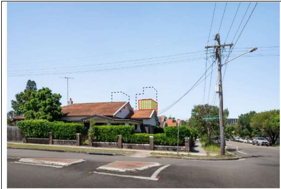
Figure 34: View from Cottenham Avenue and Day
