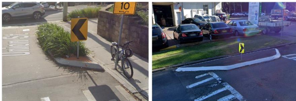
Figure 12.2: Kerb Blisters – Landscaping (left) and Standard (right)
