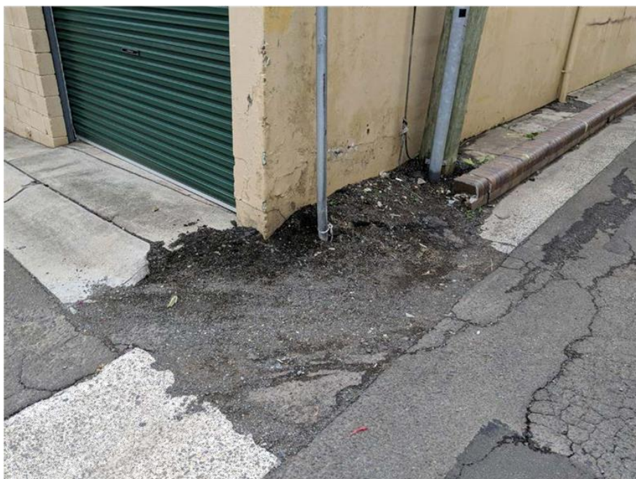
Figure 5.2: Kerb Runover at Farrow Lane
