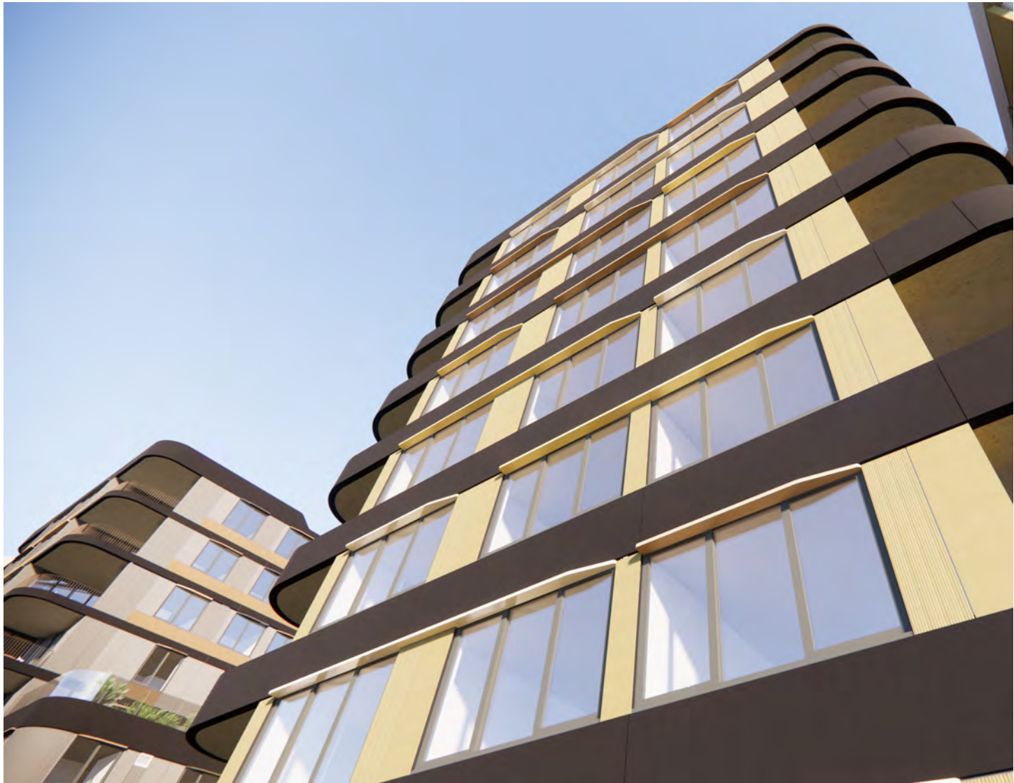
PROPOSED DESIGN - HORIZONTAL SUN-SHADING ADDED TO ALL NORTH FACING FACADES. SHADING TO PROJECT 200MM FROM FACADE AND COMPRISE CONTINOUS METAL PROJECTIONS THAT SPAN ACROSS BOTH GLAZED AND SOLID ELEMENTS OF FACADE, COLOUR MATCHED TO LIGHTWEIGHT CLADDING
