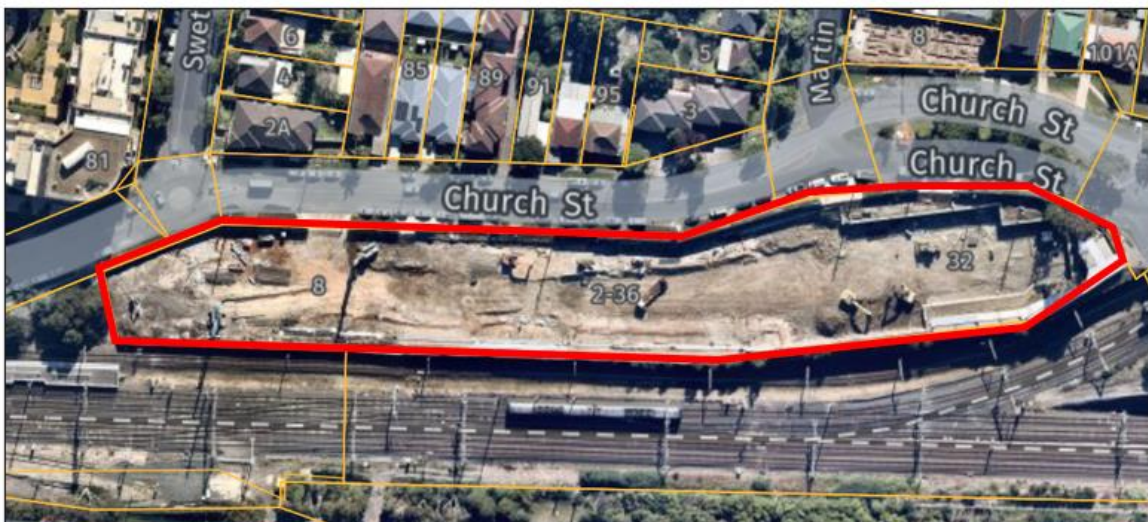
Figure 1: The Site (Source: Nearmap, 2021)
