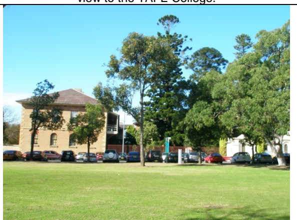
The Kurrajongs, Swamp Mahogany and Angophora along the College street boundary also partly obscure these early colonial buildings
