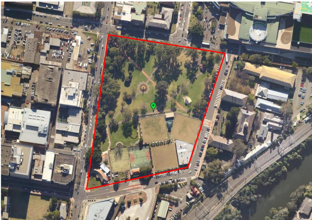
Figure 2 Aerial photograph showing Bigge Park (edged red) in the context of Liverpool CBD. (Source: Liverpool City Council)
