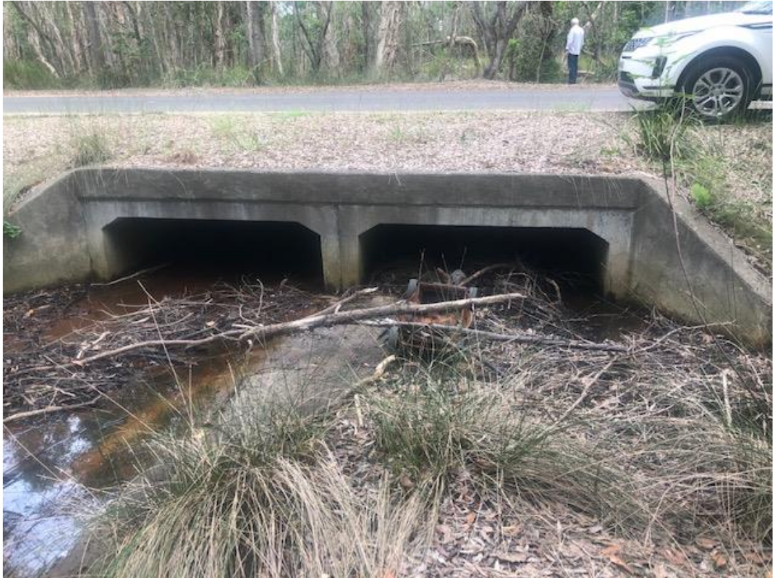
Figure 2-2 Iron Gates Drive Stormwater Culverts
