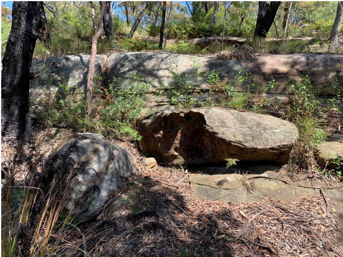
Photograph 4: View looking west, large detached block on slope suspect previous fall
