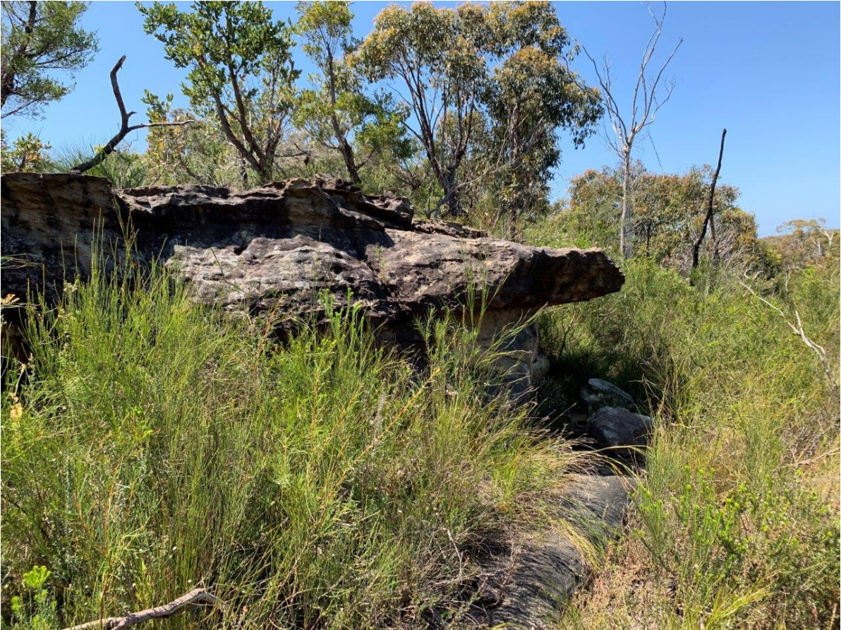
Photograph 5: View looking east, overhangs up to 1m observed in precipices up to 1.5m height
