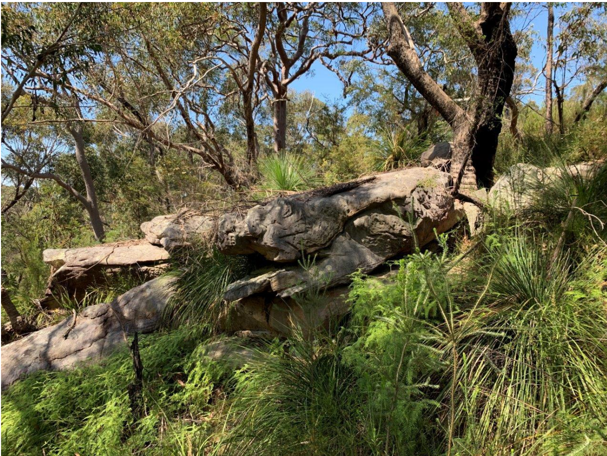
Photograph 8: View of loose block at crest, approximately 2m x 0.5m
