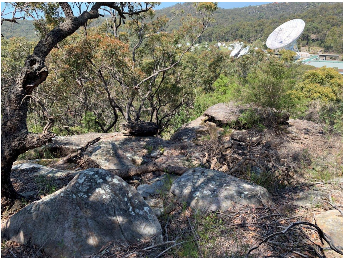
Photograph 4: View looking south, loose blocks along crest, Telstra satellite station noted in background
