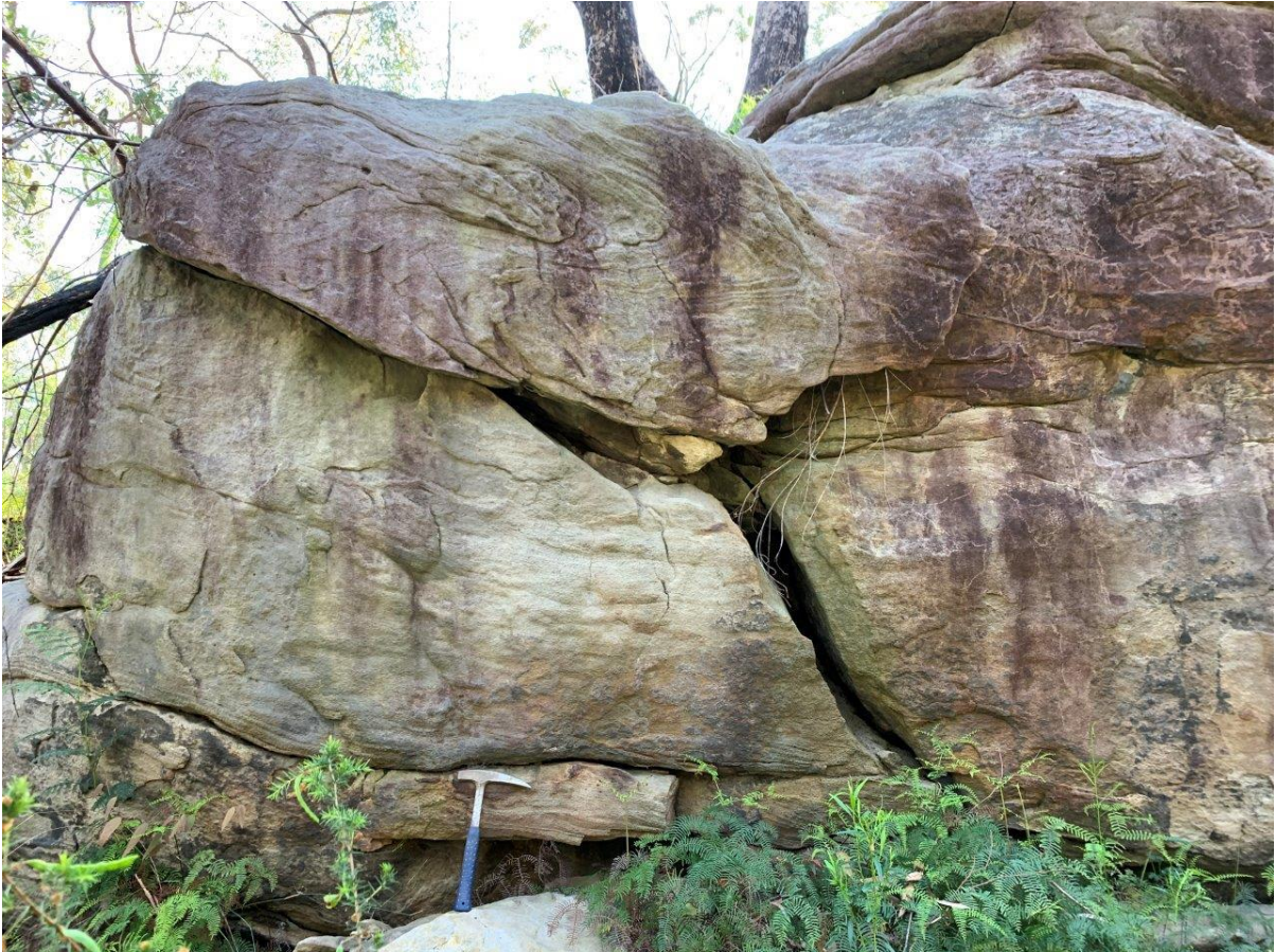
Photograph 15: View of open cracks within sandstone face, potential of fall/topple
