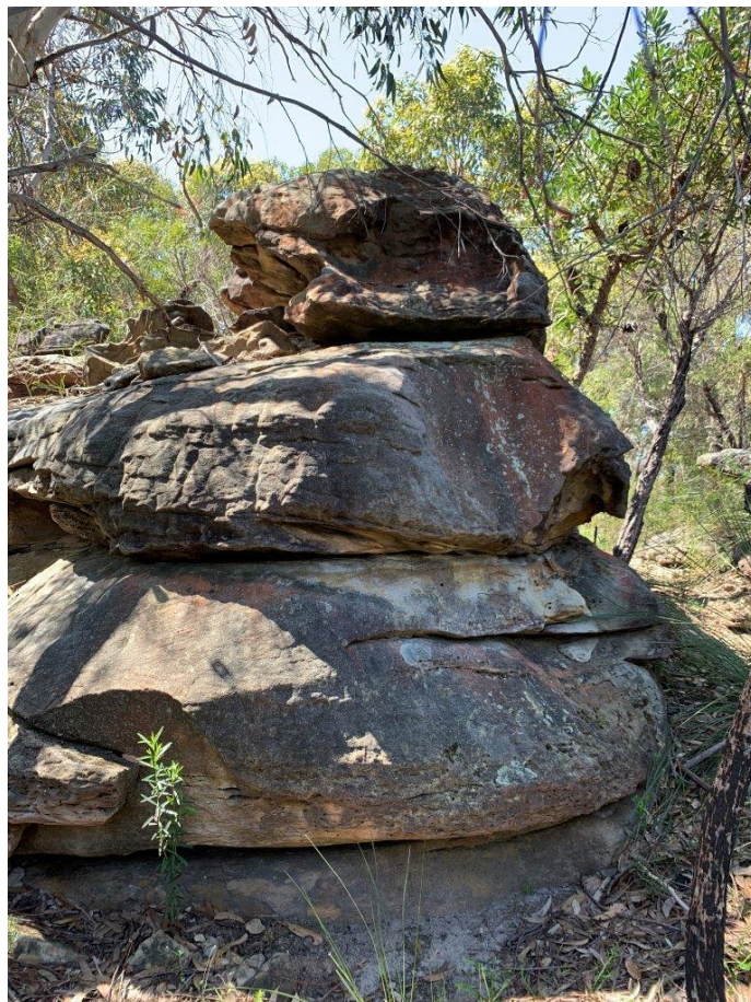
Photograph 8: View of large loose block at crest of 2m high precipice
