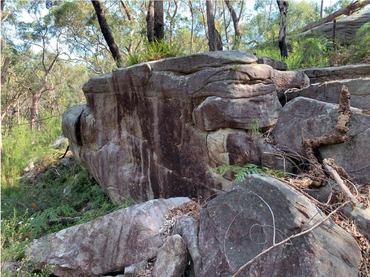
Photograph 13: View looking north-east at face of precipice, high potential of topple failure with large void behind face
