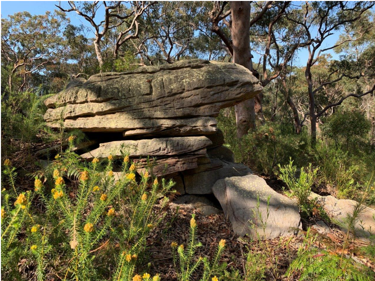
Photograph 6: View of overhangs and loose blocks on slope
