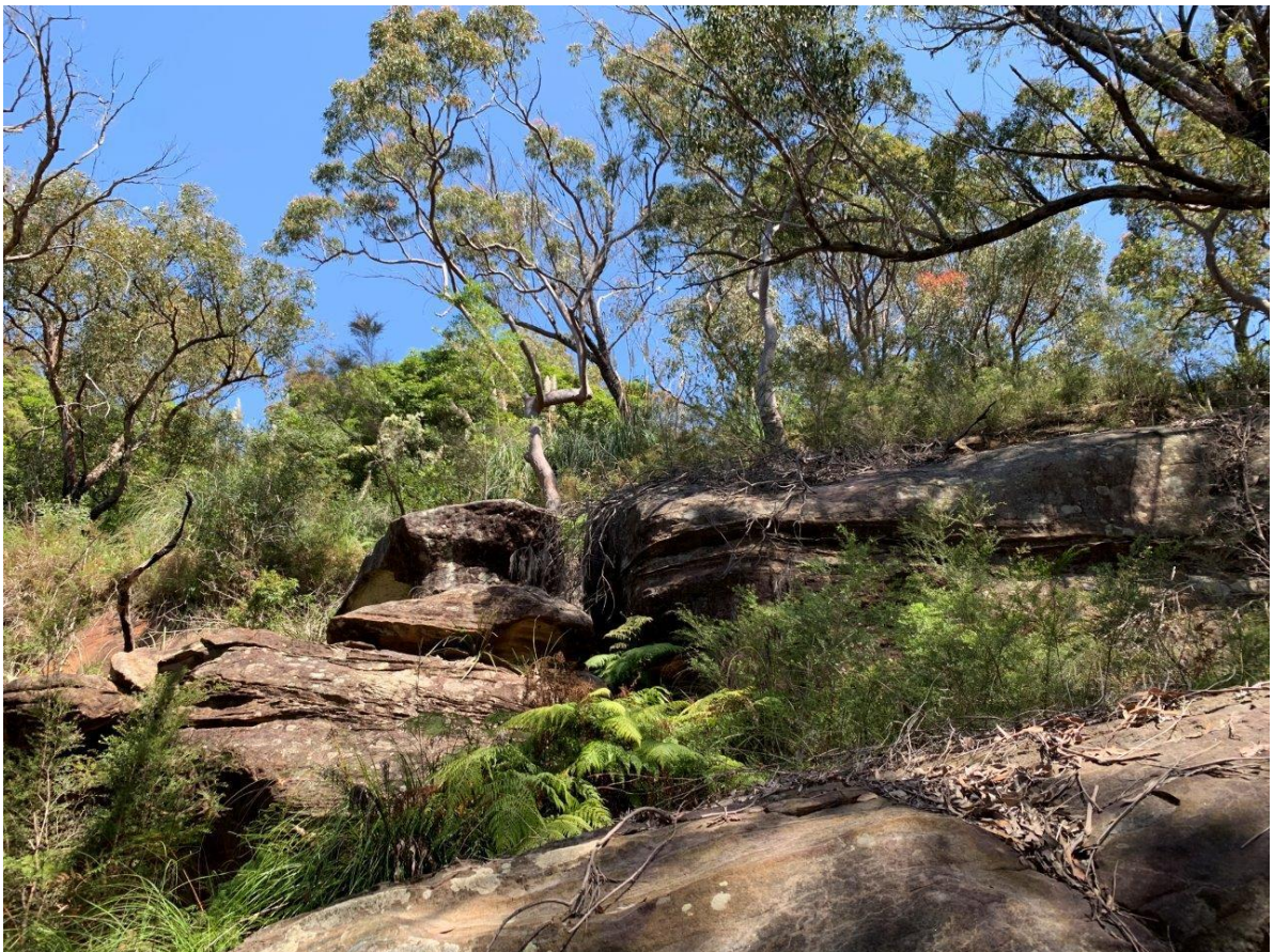
Photograph 6: View looking west, loose blocks on slope crest up to 0.8m
