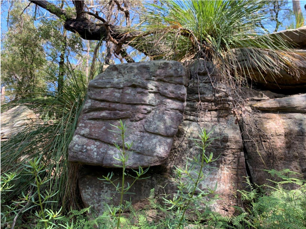
Photograph 3: View of large block, potential for collapse
