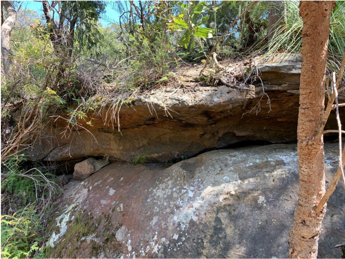
Photograph 1: Looking south, overhangs up to 0.8m observed
