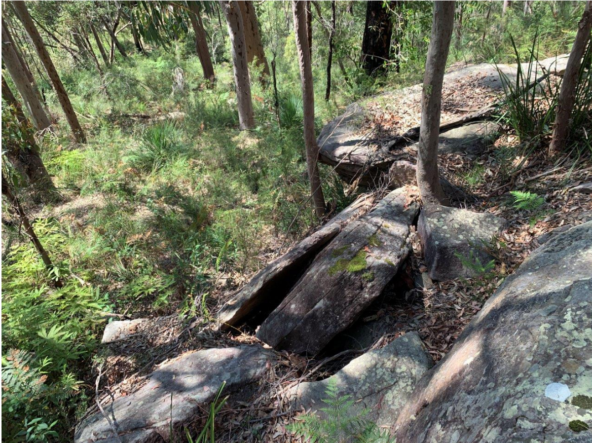
Photograph 11: View looking east, previous fallen blocks at toe, up to 0.6m
