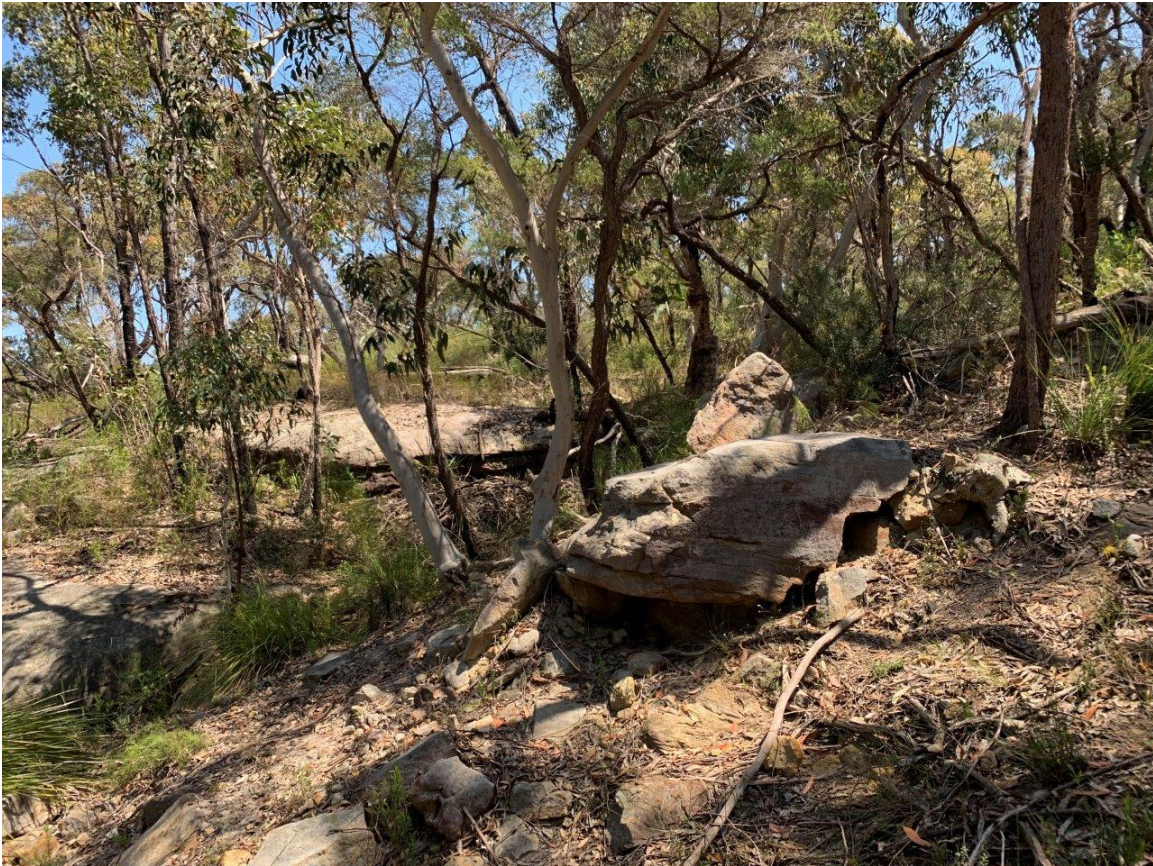
Photograph 1: View looking west, loose blocks on slope
