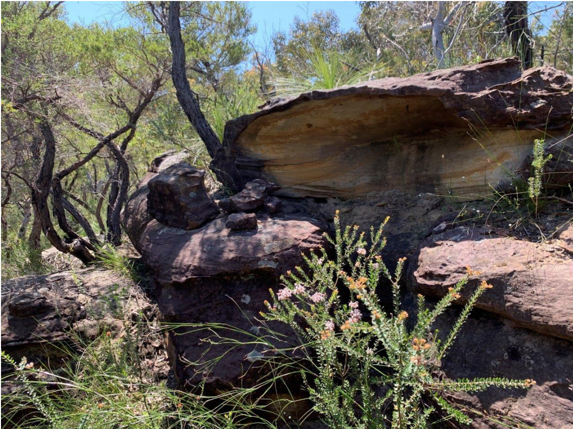
Photograph 2: View of overhangs and loose blocks at crest
