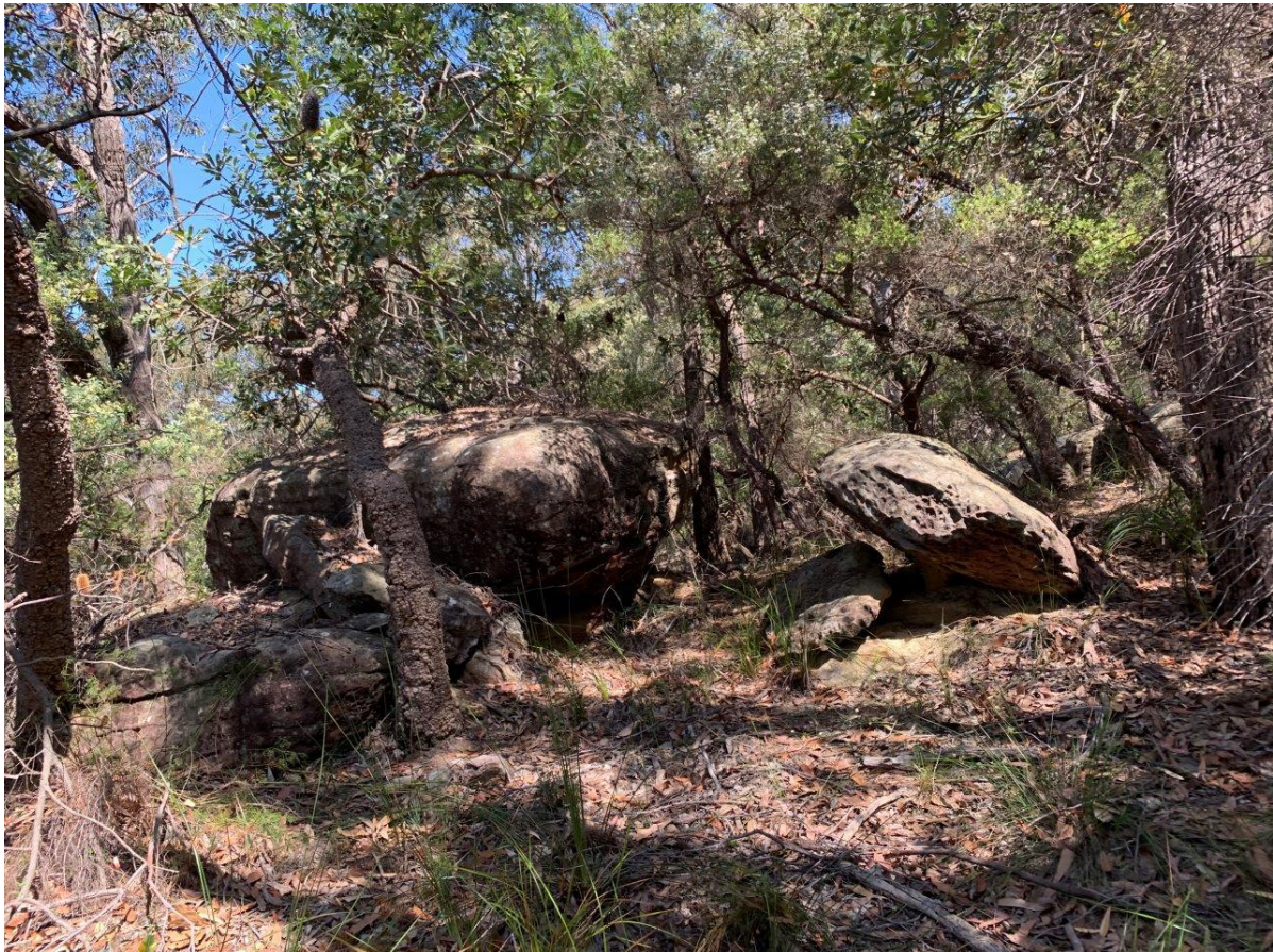
Photograph 4: View looking south-east, large loose blocks on slope
