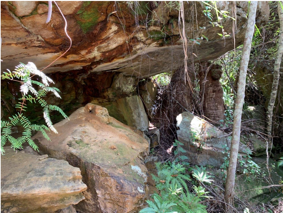
Photograph 4: View underneath large sandstone bed, loose fallen blocks underneath
