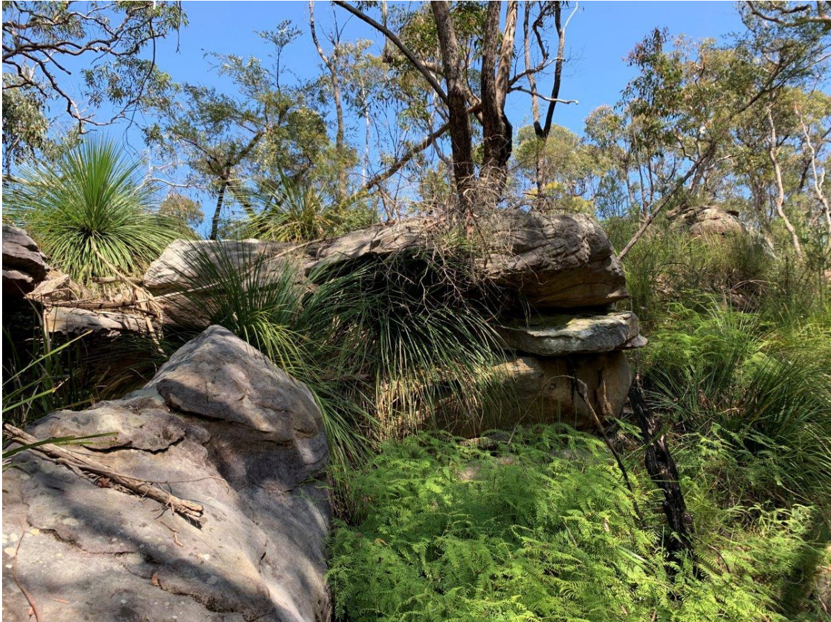
Photograph 9: View looking west, loose blocks and overhangs at crest
