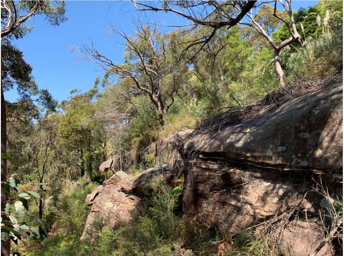
Photograph 5: View looking south along crest of precipice, large fallen blocks up to 2.5m observed
