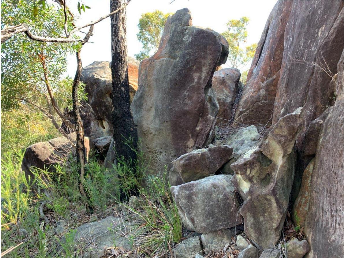
Photograph 5: View of previous falls up to 2m
