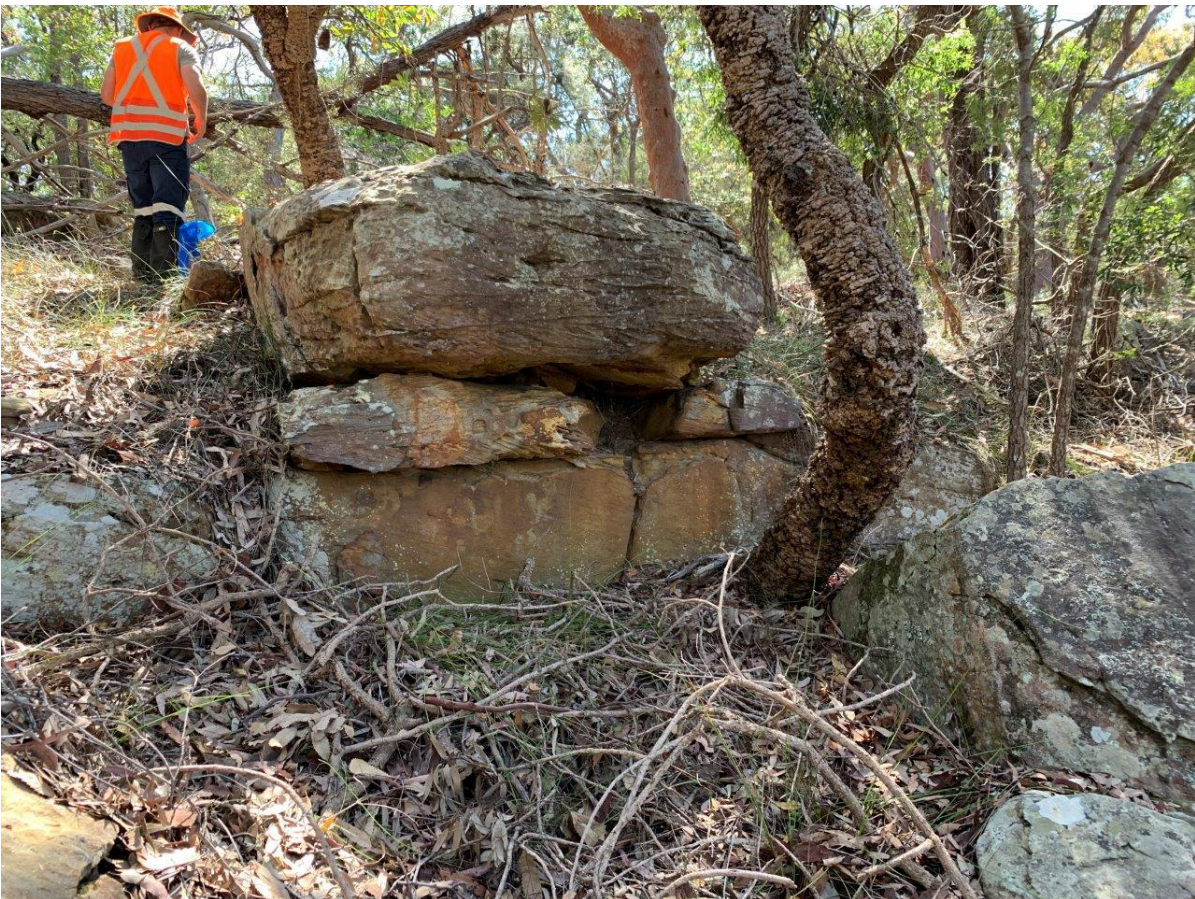
Photograph 8: View looking north, loose undercut block on slope
