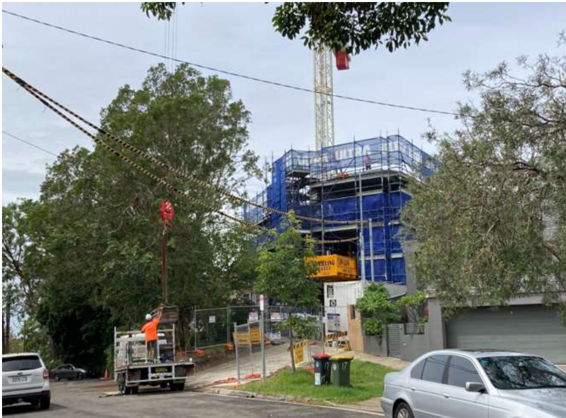
Figure 4: Apartments under construction at 21-23 Riddell Street, viewed from street.
