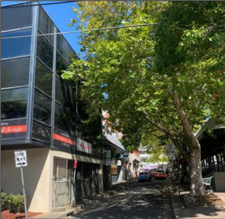
Figure 8 View of western elevation of existing site (source: Central Element)
