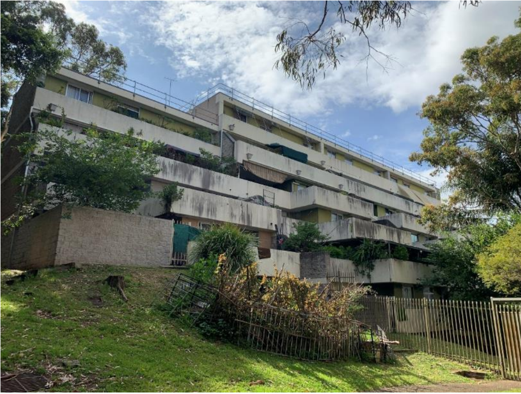
Figure 9 The Dobell building, rear facing John Street
