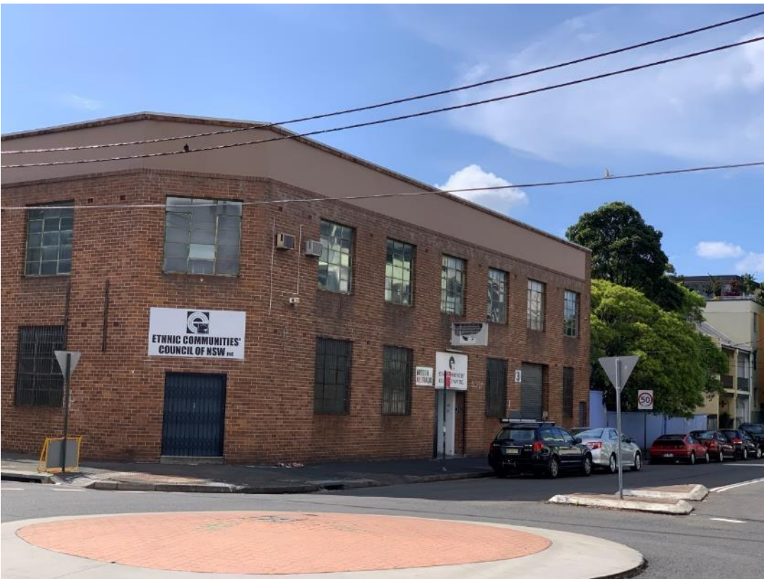
Figure 16 Commercial office building at 221-223 Cope Street
