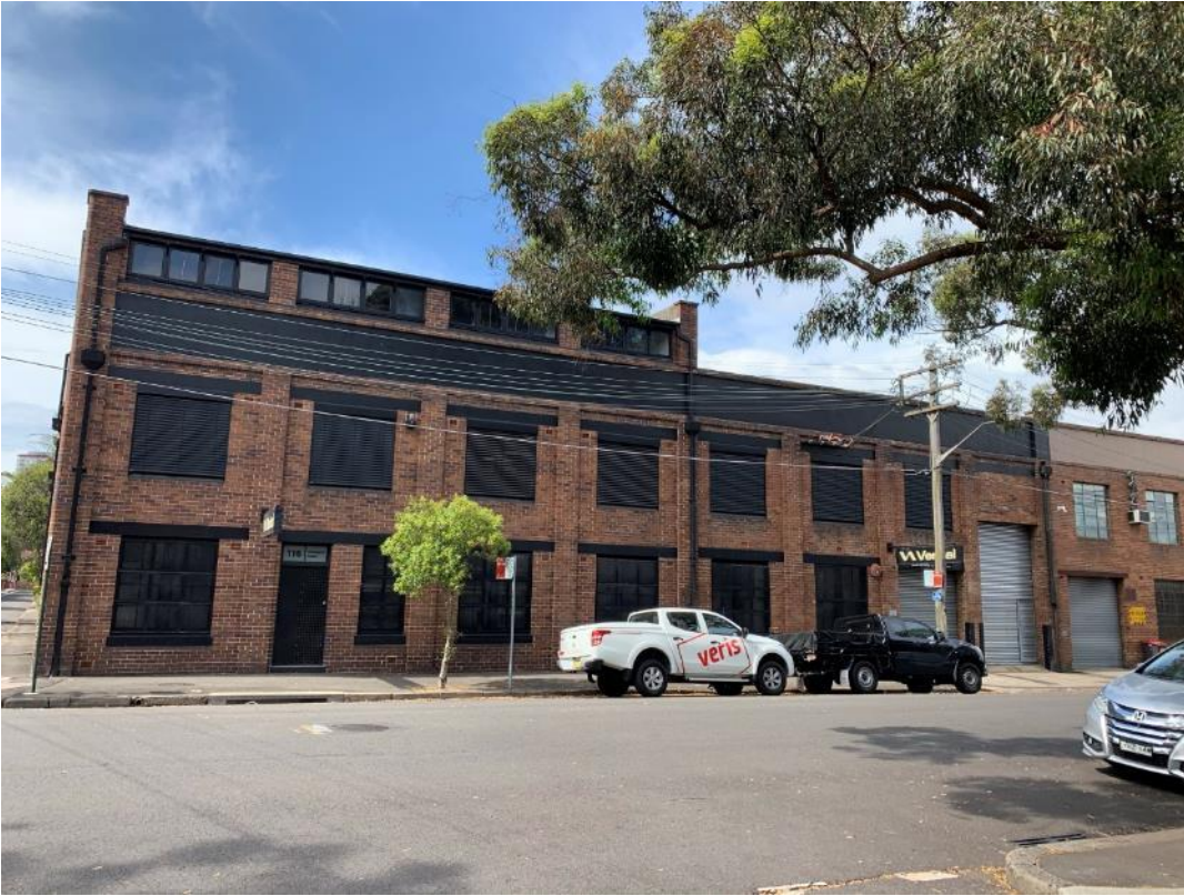
Figure 17 Industrial warehouse building at 116 Wellington Street
