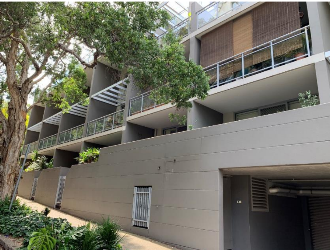
Figure 14 Private strata residential building at 110 Wellington Street
