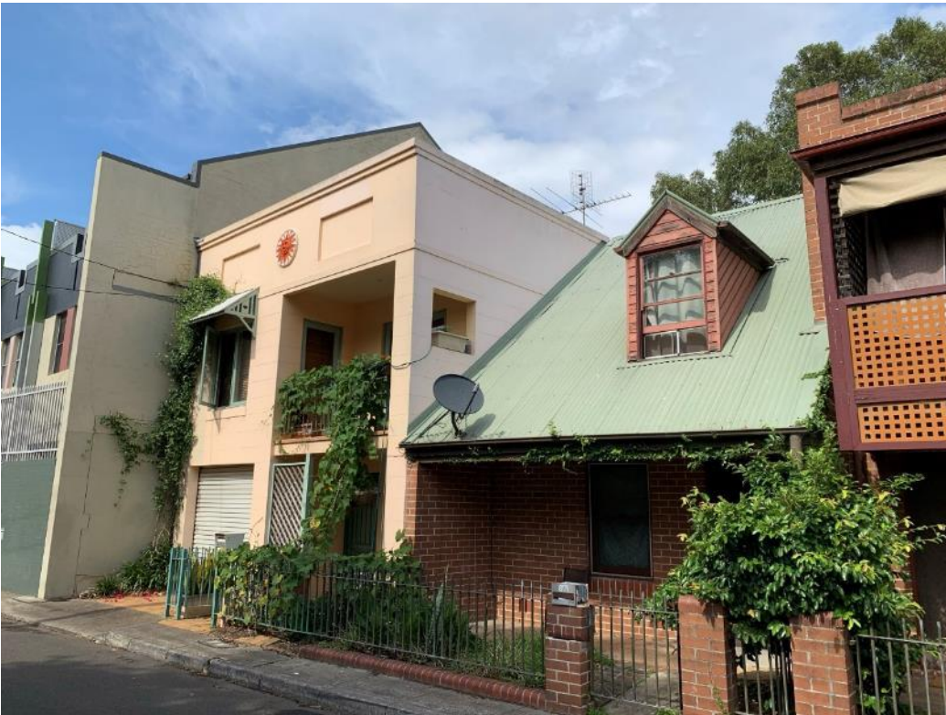
Figure 18 A privately owned terrace at 111 Cooper Street, left (the single storey house on the right is a LAHC property)
