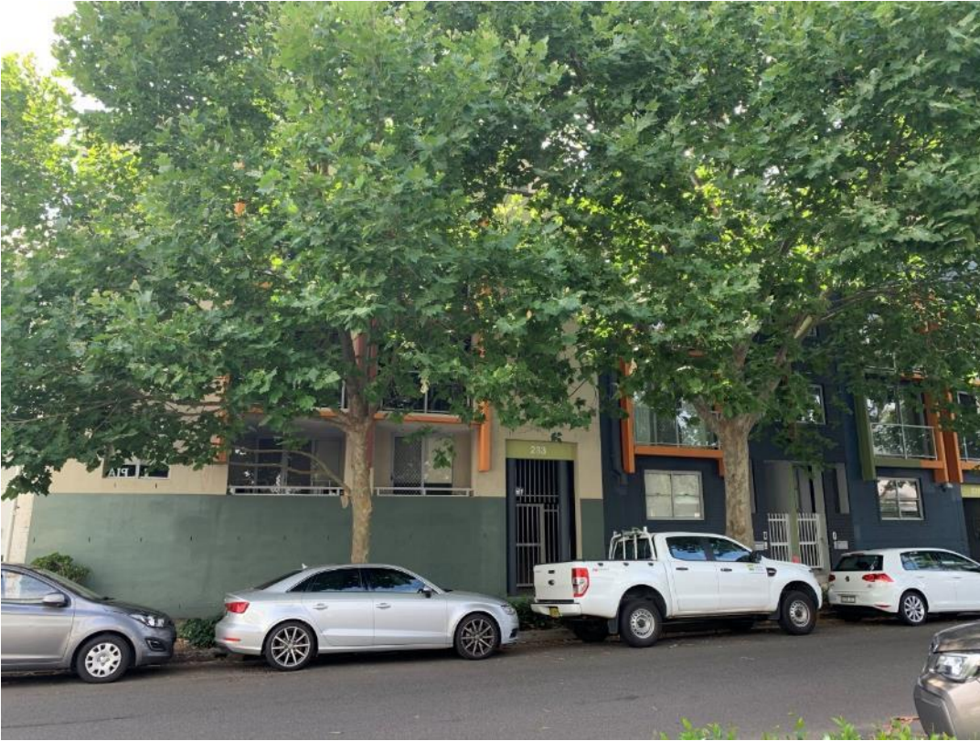
Figure 13 Private strata residential buildings on Cope Street
