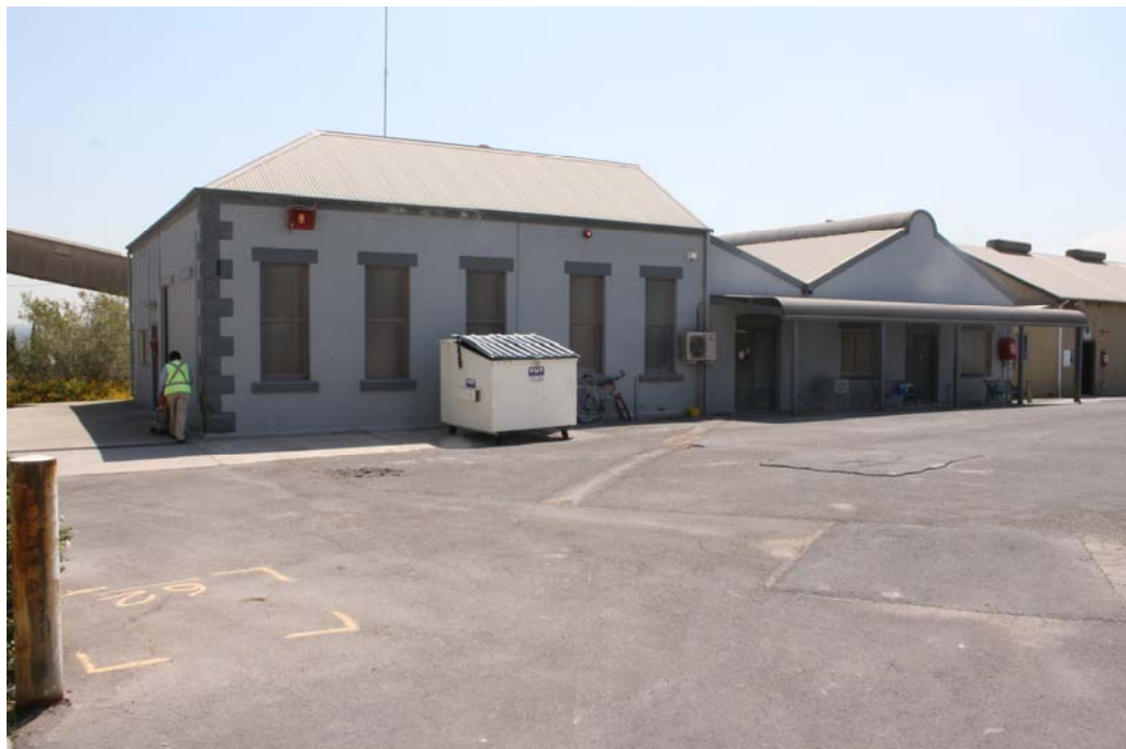
Photograph 3.1 Eastern façade of sandstone and brick building
