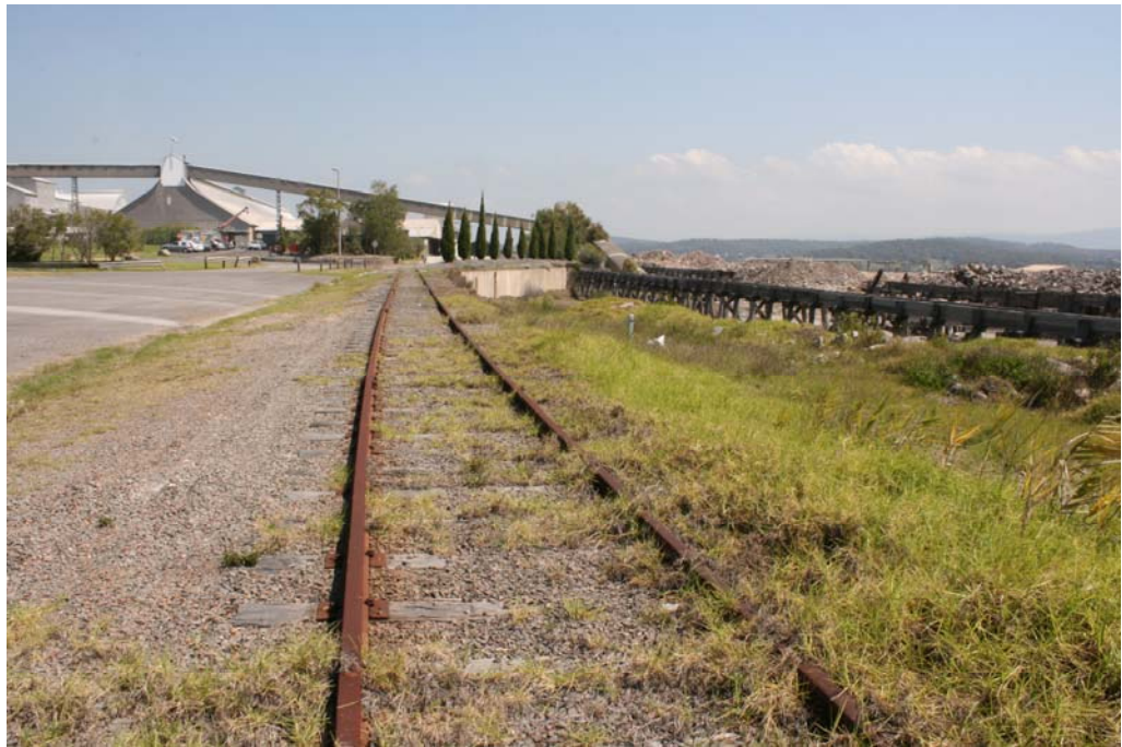
Photograph 3.6 Railway line running South West.
