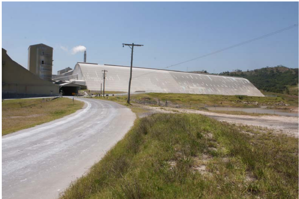
Photograph 3.4 Shed 3 (right) with end of Shed 2 on left.
