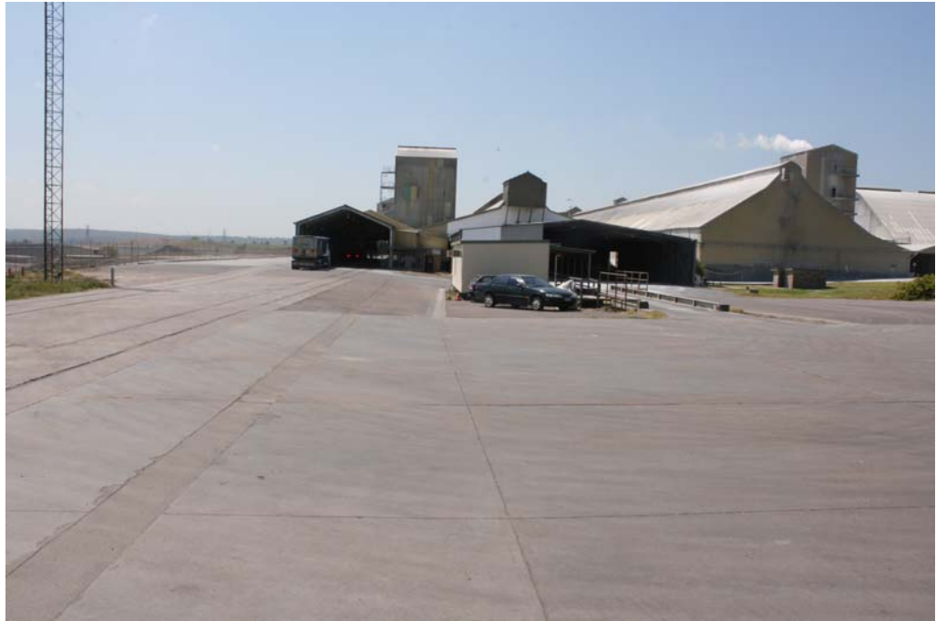
Photograph 3.3 Shed 1 (left) and Shed 2 (right) with railway line running through Shed 1.
