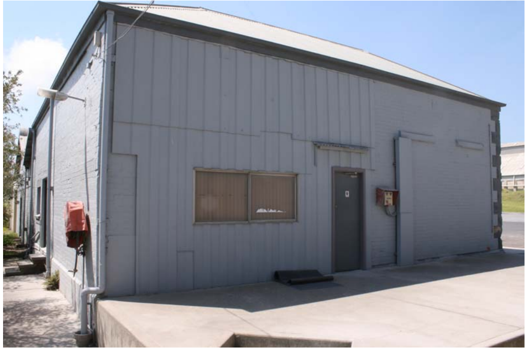
Photograph 3.2 Southern façade of sandstone and brick building
