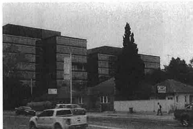
Figure 6 – Development to the south of the site
