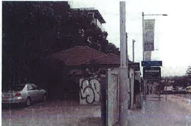
Figure 4 – The site, as viewed from the western side of Lane Cove Road
