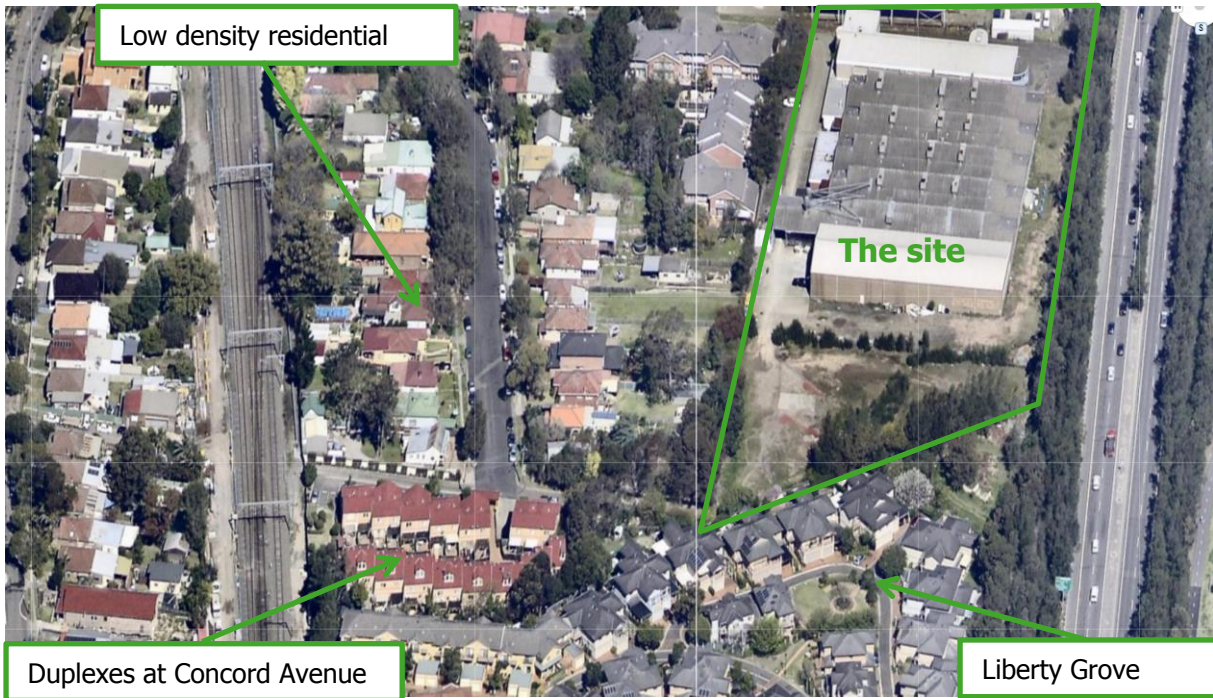
Figure 13 Aerial view of site and surrounds facing south
