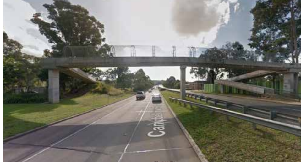
Open space continues further SE of the site across Campbelltown Road
