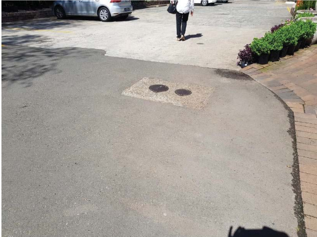
G: Photograph of disused UST within nursery carpark and monitoring well (MW1) in the background
