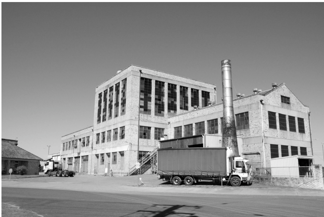
Figure 4.2 Former Peters Dairy Factory, 2007
