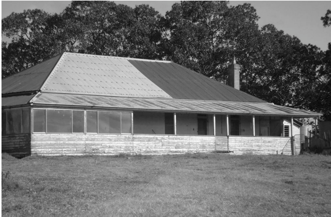
Figure 1.1 Small house at Swan Creek, 2007
