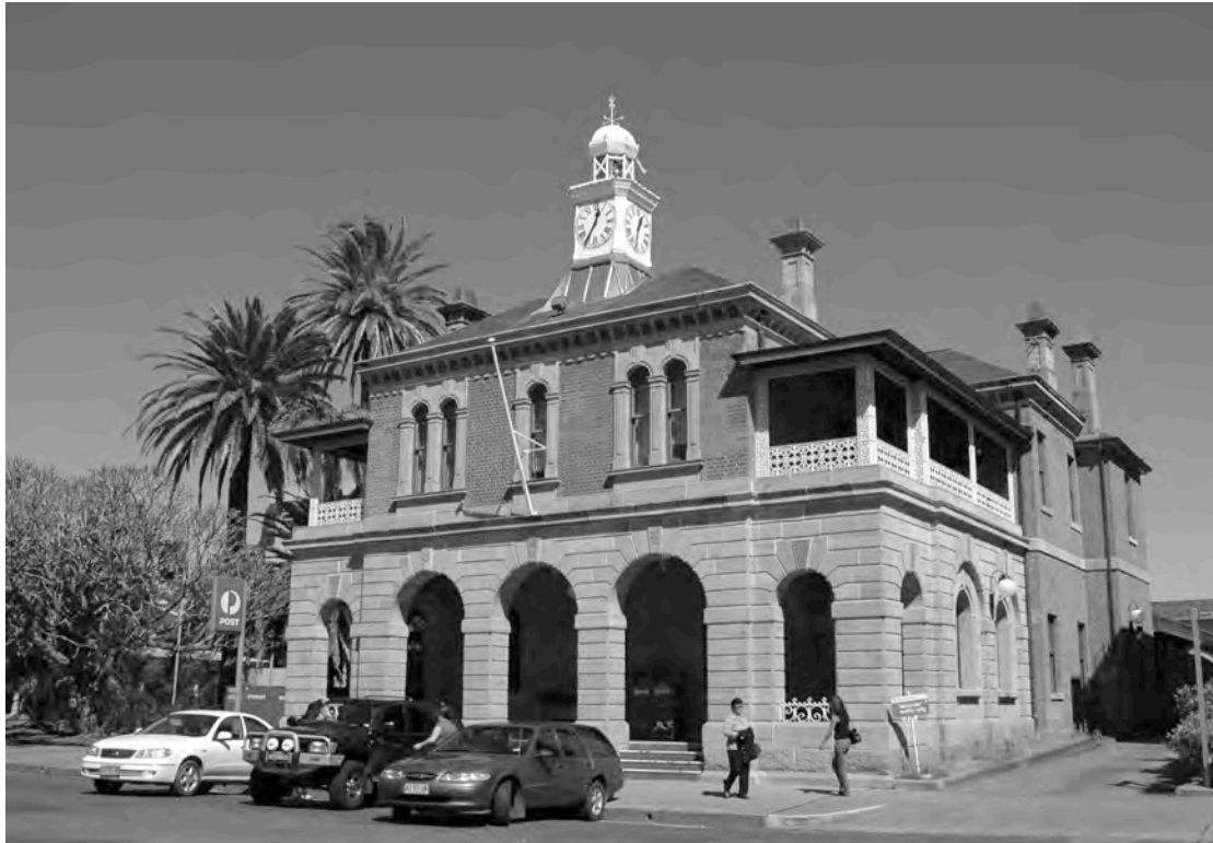
Figure 3.1 Grafton Post Office, erected 1874-1877 and opened 1878.
