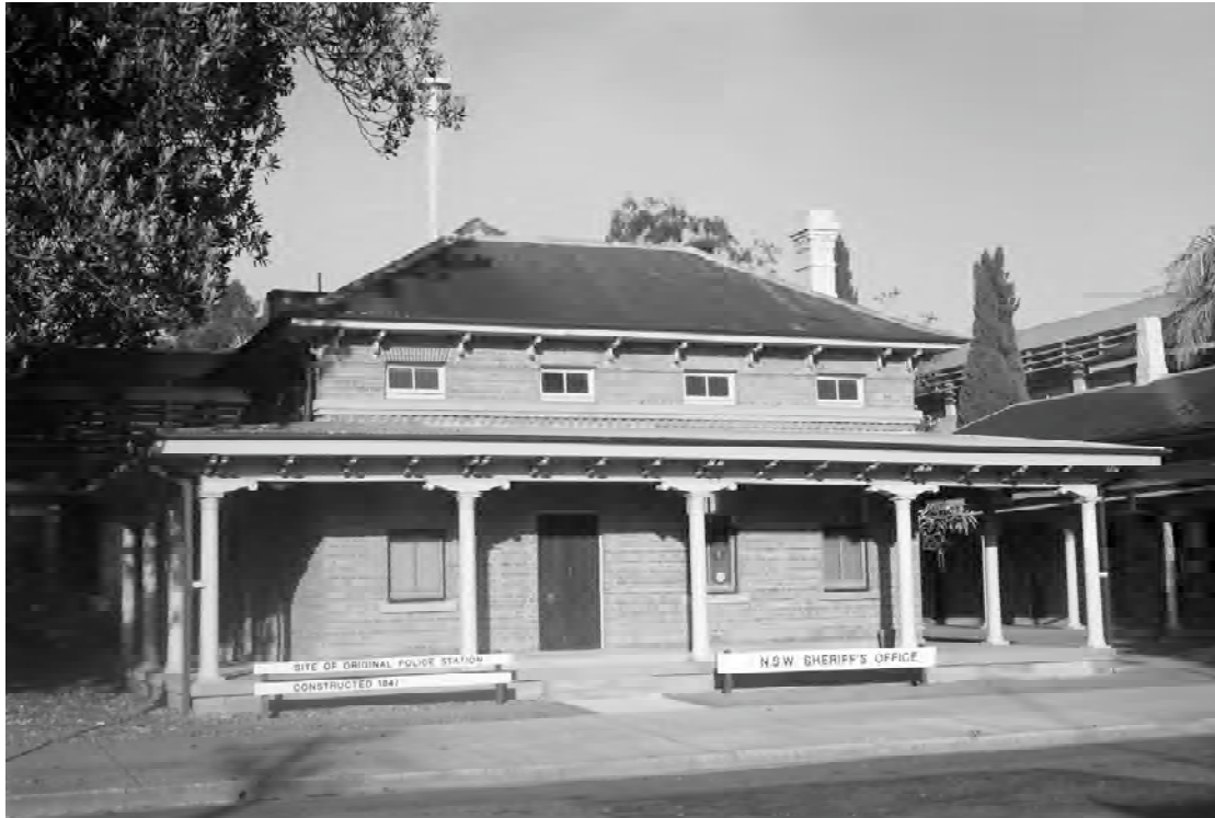
Figure 2.2 Former Grafton Court House, 2007. This structure is the 1880s extension to the second (1861) court house, the ruins of which adjoin it at the rear. The sign erroneously states that this is the 'site of [the] original police station constructed 1847'.
