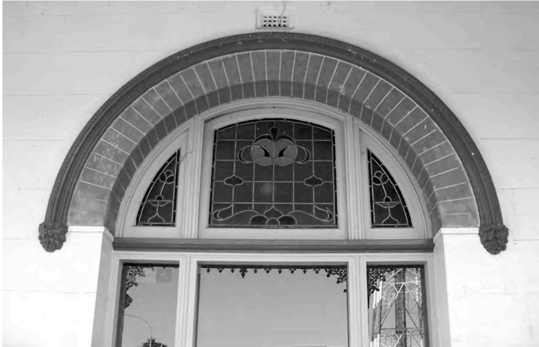
Figure 2.10 Window detail, former Weiley's Hotel, Prince Street, Grafton, 2006
