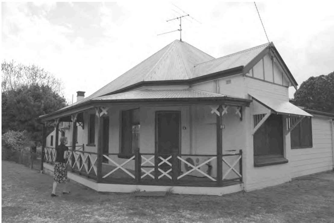
Figure 2.8 Former Vineyard Hotel, 2007. Although this building was licensed as a public house for only about ten years, it is interesting because of its age (erected c.1869) and its connection with Grafton's German community (its first licensee was Philip Hoffman). It is one of the oldest surviving pub buildings in the city.
