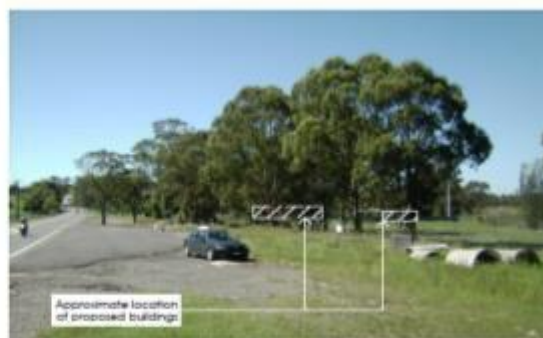
Figure 6 – View northbound along Campbelltown Road
