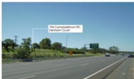
Figure 7 – View northbound along M5 Motorway
