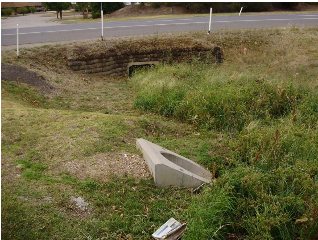
Donnolley Court Drainage Reserve and culvert looking North towards Wagga Road
