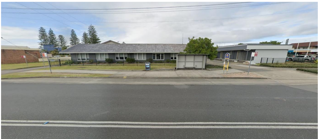
FIGURE 2.9: BUS STOP IN BEACH STREET 150M NORTH OF SITE PHOTOGRAPH SOURCE: GOOGLE STREET VIEW IMAGE CAPTURE MAY 2018
