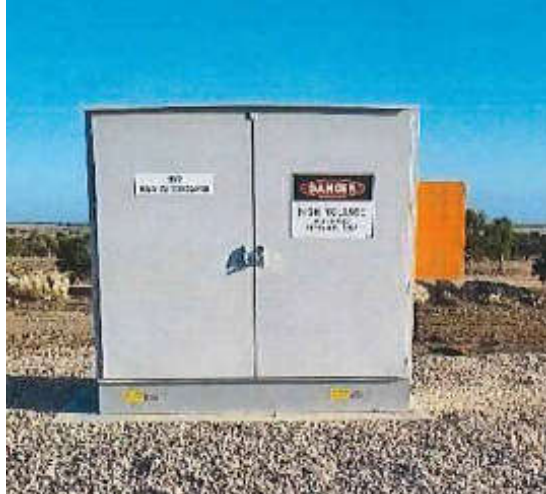
Figure 5 – Image of a typical Ring Main Unit (RMU) (image taken from SEE)
